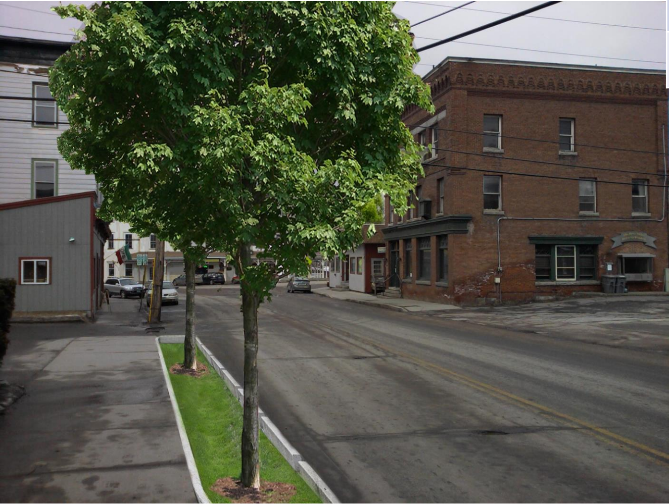
C.1. Grass-and-tree vegetated bioretention cell with curb cuts to capture and filter stormwater using plants and soil.
