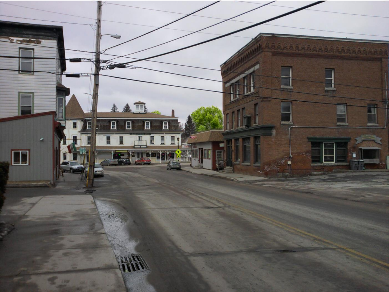
A.1. Conventional stormwater infrastructure with drainage grate, catch basin, and storm pipe directing runoff to storm sewer.
