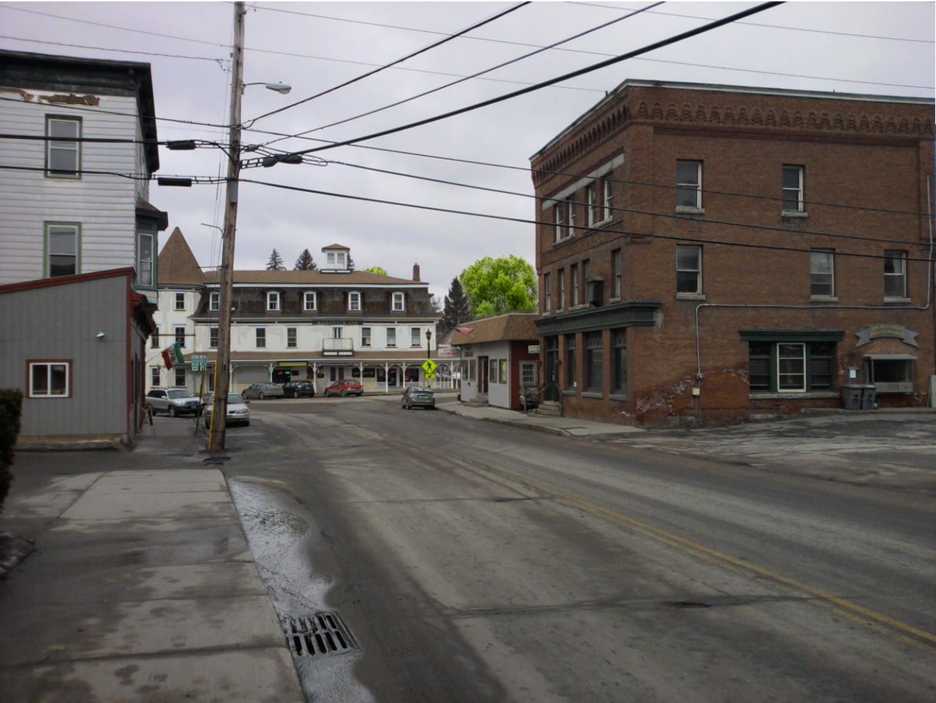
A.1. Conventional stormwater infrastructure with drainage grate, catch basin, and storm pipe directing runoff to storm sewer.
