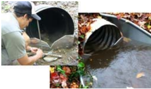
Figure 3: Photos showing (upper left) installation of double v-notch weir and suction strainer at culvert inlet and (right) flow over the weir during a storm event.
