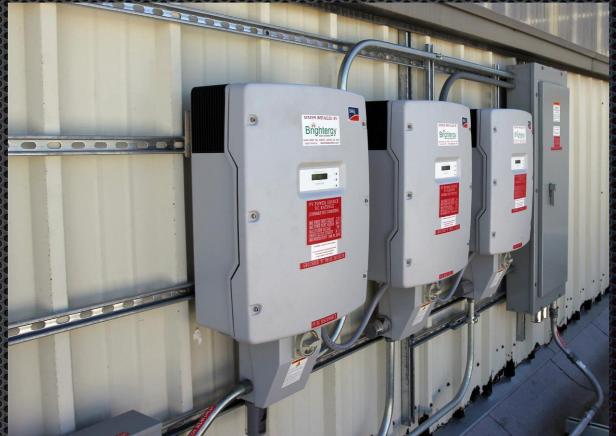
A series of solar inverters ( brightergy.com )
