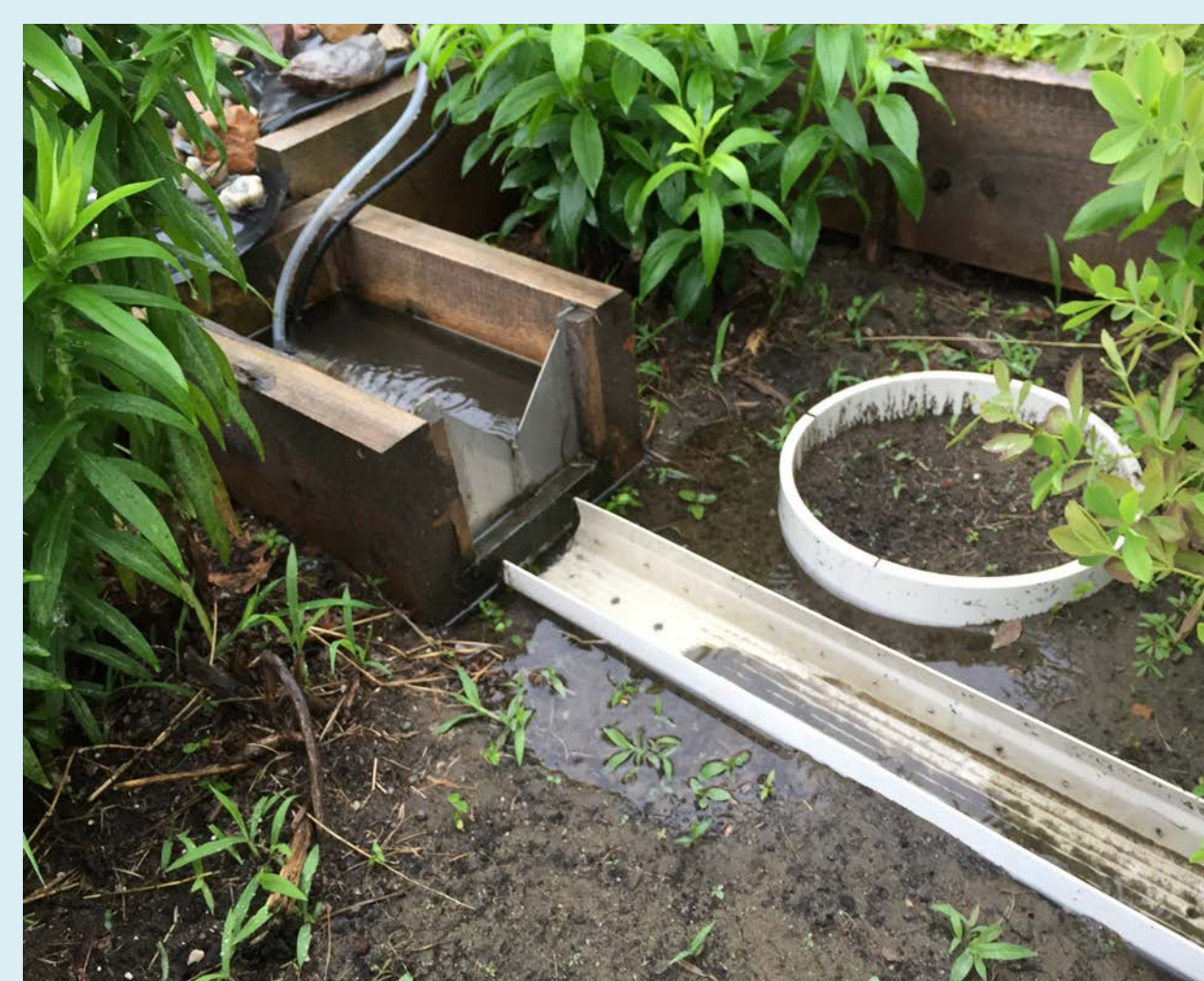
Figure 2 – Flooded Bioretention Basin
