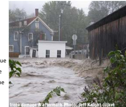
Photo: Damage to a home after photo: Jeff Magid, @jeff
