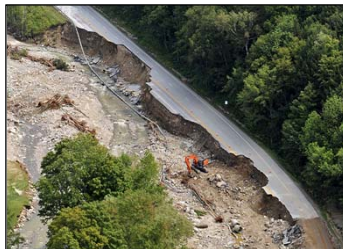
Mad River Valley Flooding Damage During Hurricane Irene Image Source: VT Agency of Natural Resources
